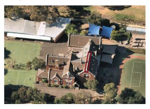
To allow for the flashing to be installed, the ridge capping was lifted and reinstated with the existing fixings. On Wednesday 26<sup>th</sup> of April, a length of ridge fell from the roof onto the garden bed area below. A make safe was carried out after hours to ensure the remaining sections of ridge cap were secure and we found that the head and thread of the screws used to secure the ridge cap had failed.
